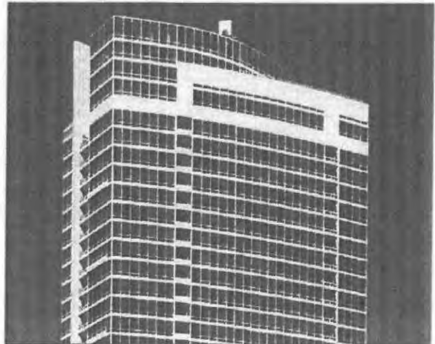
Streeter Place Location: Chicago, IL Product: Solarban 60 Glass Architect: Solomon Cordwell Buenz and Associates Owner/Developer: Golub and Company Glass Fabricator: Northwestern Industries, Inc. Glazing Contractor: Custom Windows and J&D Erectors
